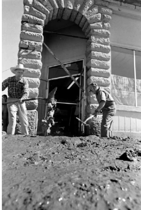
ADVANCE FOR RELEASE SATURDAY, JUNE 11, 2016, AT 12:01 A.M. MDT. - This June 1976, photo shows people cleaning up Sugar City, Idaho after the Teton Dam collapse. Forty years after the Teton Dam collapse, many eastern Idaho residents vividly recall the chaos set in motion that sunny Saturday morning. (Robert Bower/The Idaho Post-Register via AP) MANDATORY CREDIT
